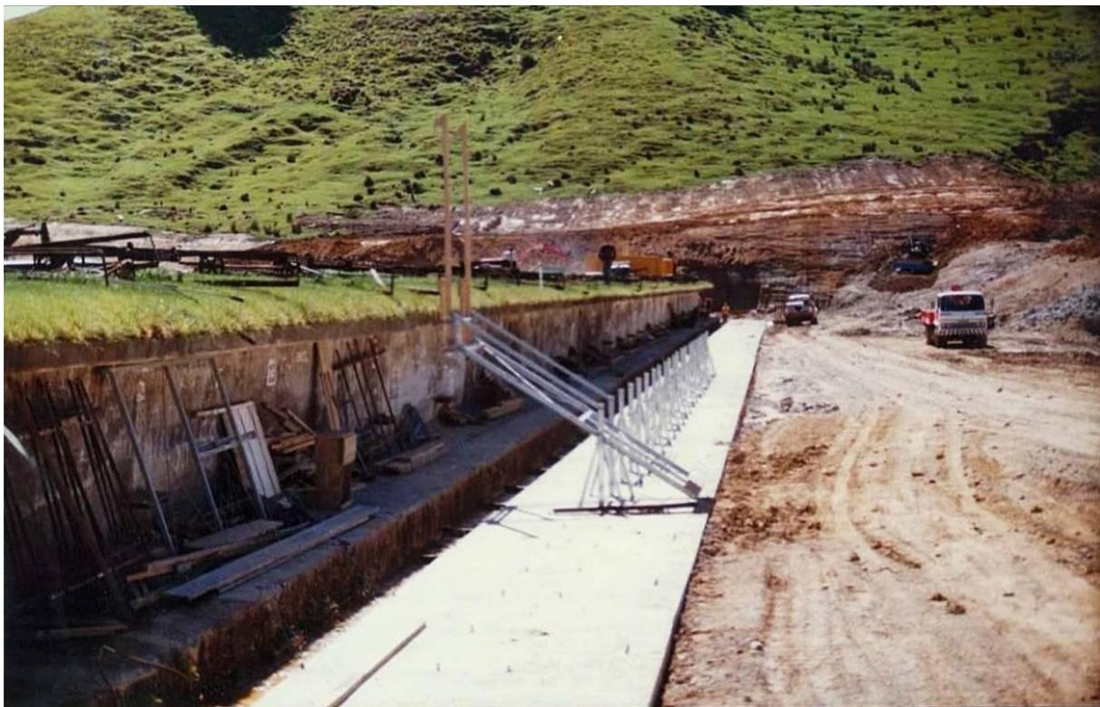
The new target hoists being erected on a new concrete platform. (NRANZ)
